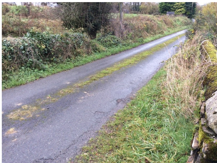
Plate 17: CH8 bridge on Proposed Grid Connection Route.
